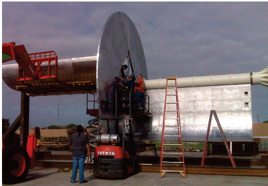
SkyDrill Full Scale Model Construction
